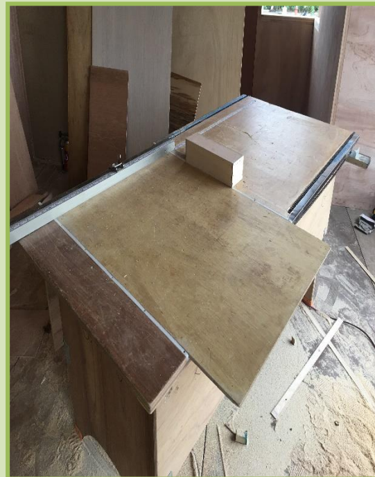
After 設置接觸預防裝置
