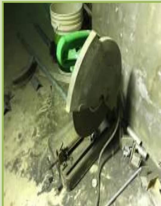
After 設置鋸齒接觸預防裝置
