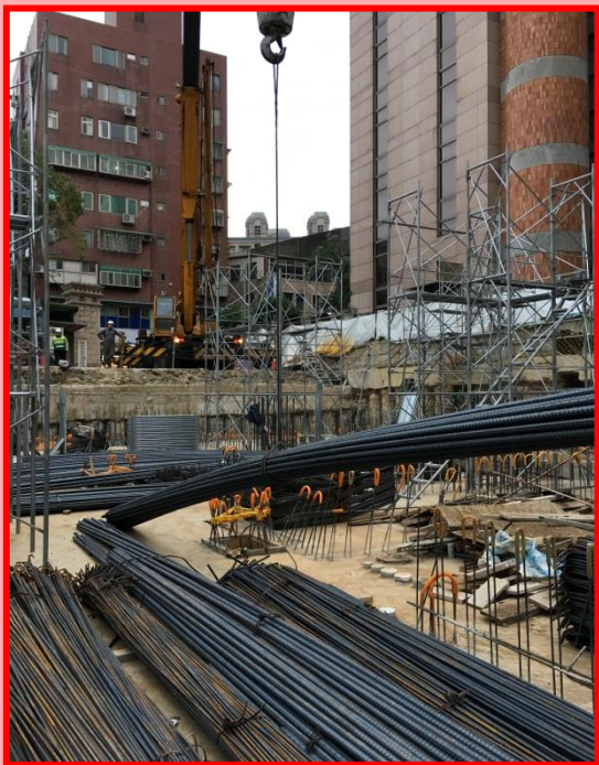
Before 僅以拉索一端捆紮吊運
