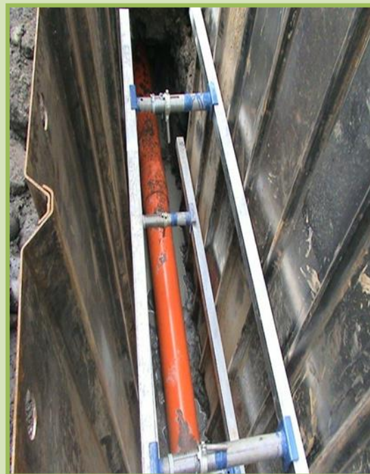
After 設置擋土支撐
