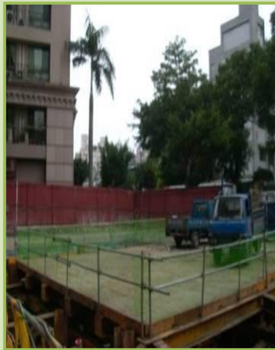
After 設置合格護欄
