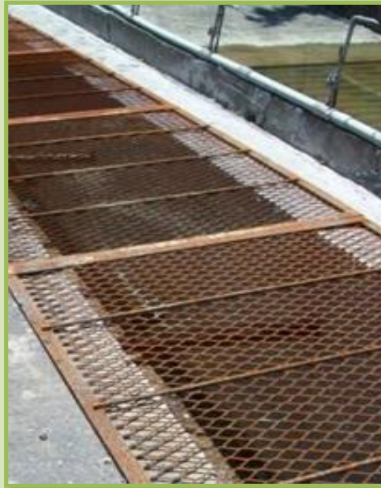
After 導溝設置護蓋
