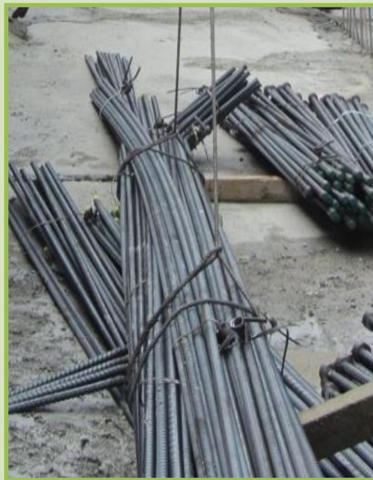
After 兩端以拉索捆紮吊運
