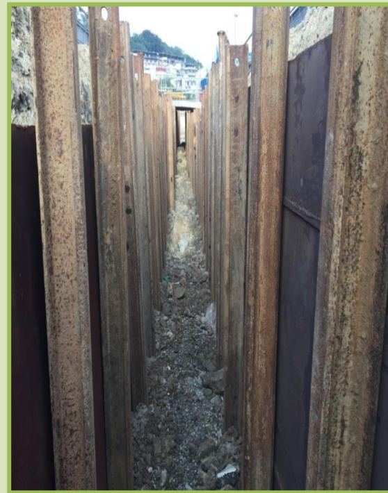
After 設置擋土支撐
