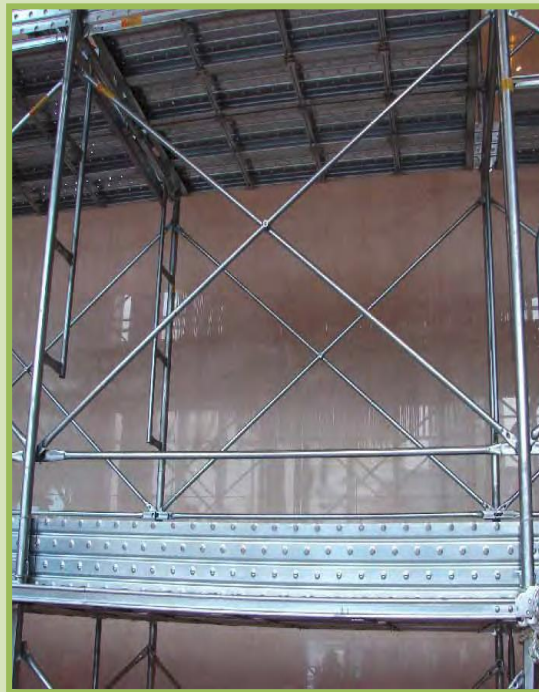
After 合格材料施工架
