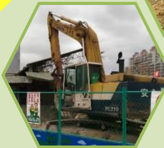
After 挖土機3大缺失改善
