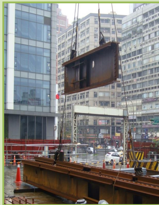
After 保持吊運構架平穩
