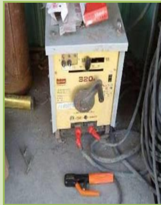
After 設置絕緣被覆
